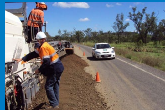
Mine Haul & Access Roads
