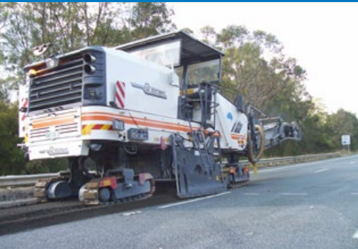
Road Profiling & Excavation
